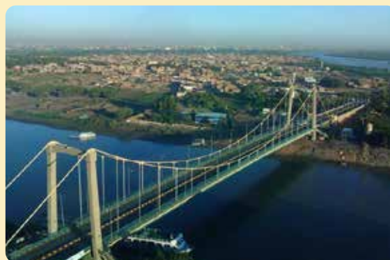
Title: Road bridge connecting Tuti Island to Khartoum Sources: http://photos.wikimapia.org/p/00/04/62/33/35_big.jpg
